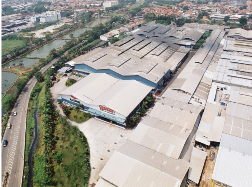
Kapuk Plant (Radiator Facilities)
